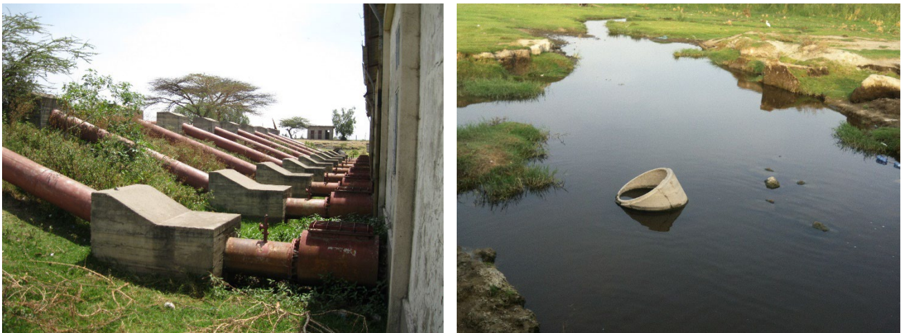
Fig. 7 and 8: Electric pumps to remove water from the lake and wastewater discharge to Lake Ziway from floriculture industries. © Hayal Desta. All rights reserved.
